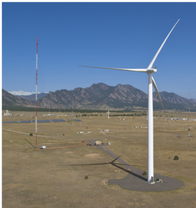
Figure 3.1: The Siemens 2.3 MW turbine at the National Wind Technology Center. The red and white trussed tower in the left portion of the figure is the M4 meteorological tower. Photo credit to Dennis Schroeder, NREL.
